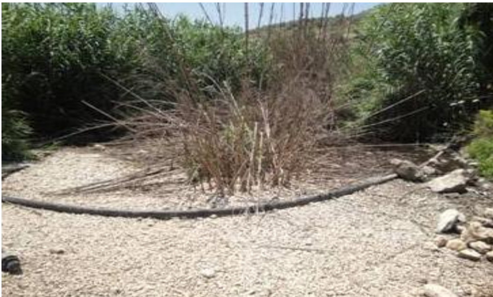
Photo 3. Reeds planted in the constructed wetland basin of Bani-Zeid pilot WWT
