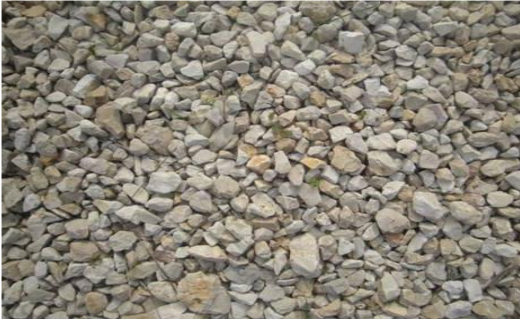
Photo 6. Gravel in the constructed wetlands basin of Bani-Zeid pilot WWTP
