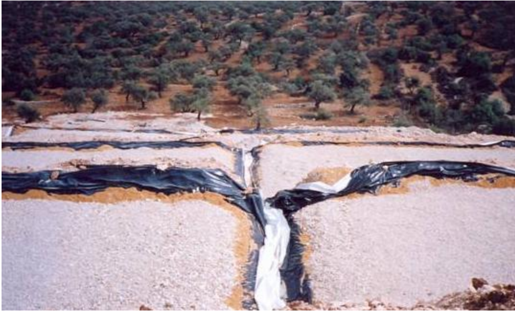
Photo 2. Wetlands construction in 2004 (Photo by PHG 2004)
